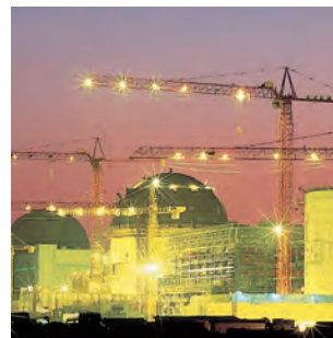
Power plant construction
