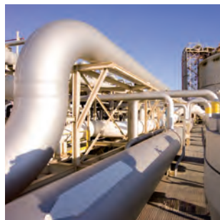
Process plant construction
