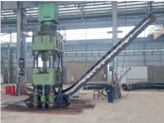
Cold bending of a large pipe.
